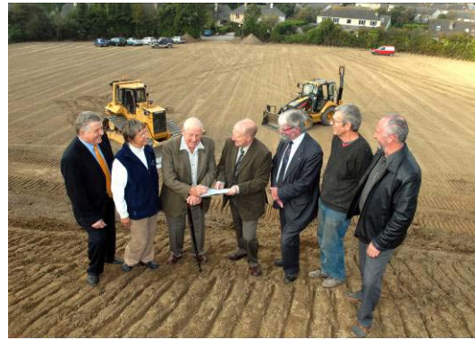
Picture by AgriMedia (Rushworthy 08/08/2007) HGCC Affordable Housing site at St. Minver. (L-R) Alan Fox (Project Manager CLT), Helen Roberts (St. Minver CLT), David Webb (Joint Mayor & St. Minver Charley Trust), Steve Cranner (Affordable Housing officer), Clr Graham Fooks-Martin (Chair HGCC), Ted Rowe (B&P contractor advisor), Richard Wilson (Trustee - Finance).
